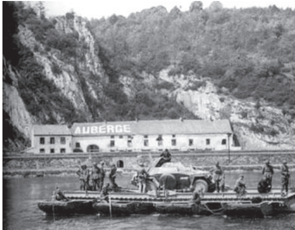
Figure 7. 1940 Meuse crossing at Auberge NARA
